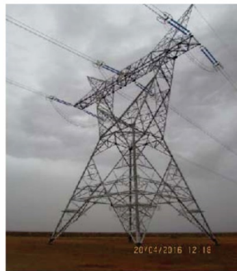
400kV 517F Tower Closing Span Tower or Angle Strain Tower Max Height: 35m Width Top: 23.2m Width Bottom: 18m
