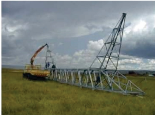
Typical example of crane
