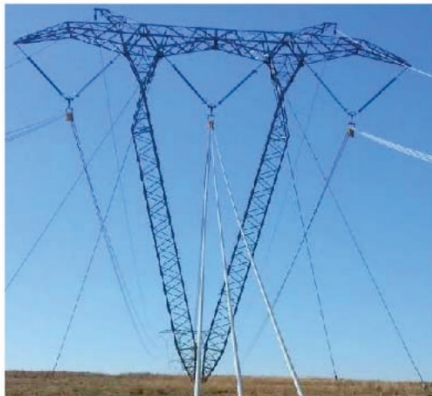
400kV Guyed Vee Suspension Tower Max Height: 40m Width Top: 23.4m Width Bottom: 1m
