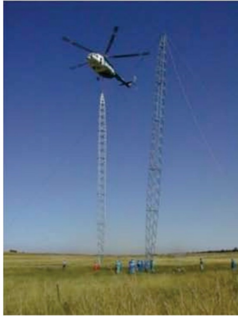
Figure 3: Typical construction equipment
